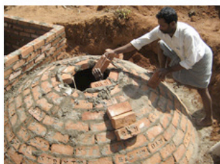
Construction of a biogas reservoir
